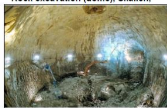
Rock excavation (dome), Skallen,
